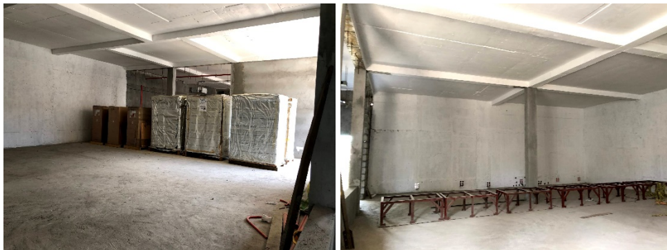
Status of new data center on Day 1 of our in-country implementation phase
