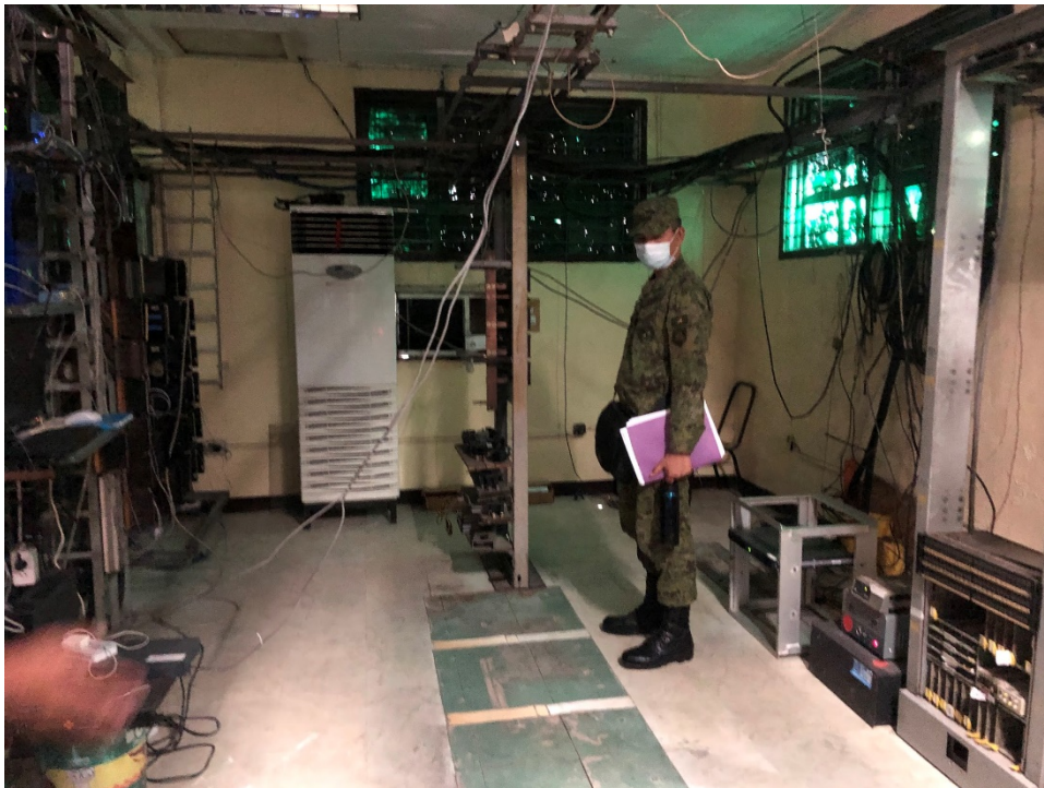
The temporary location for the data center
